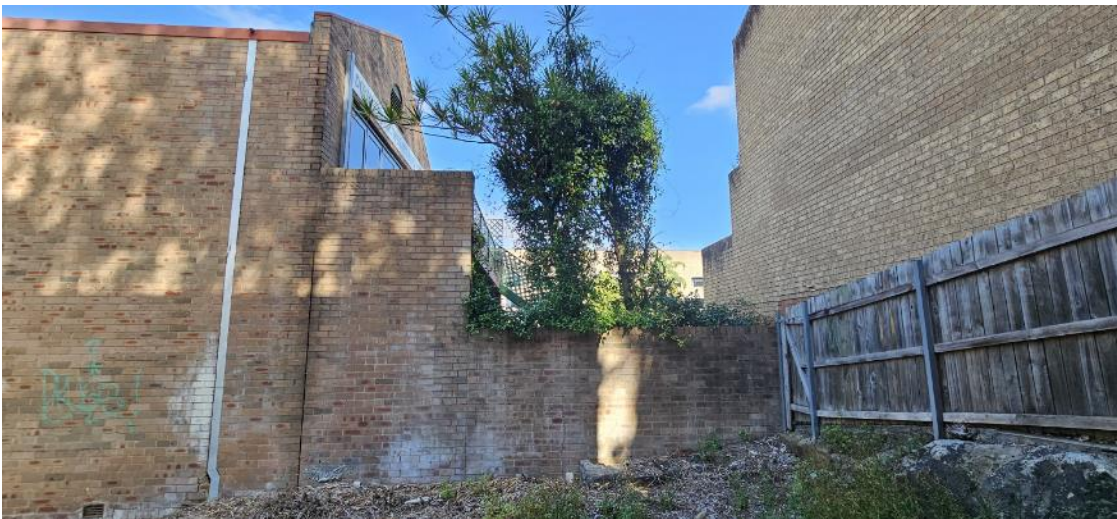
Figure 7: Adjoining building at no. 31 viewed from rear courtyard facing south
