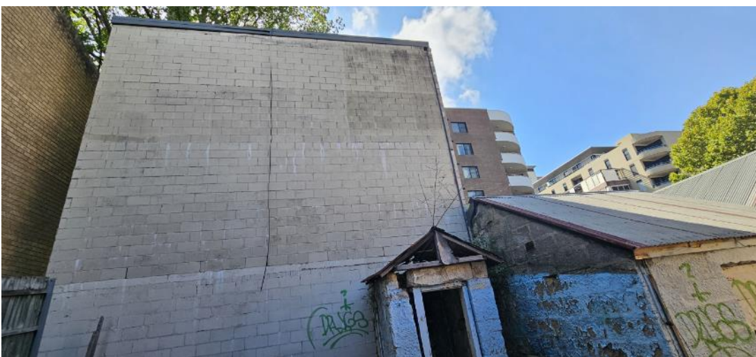
Figure 8: Adjoining building at no. 27 viewed from rear courtyard facing north
