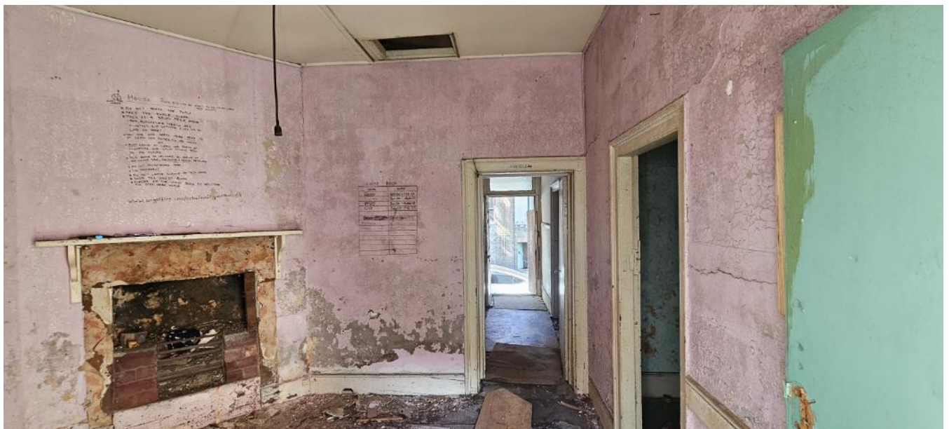
Figure 14: The rear north room
