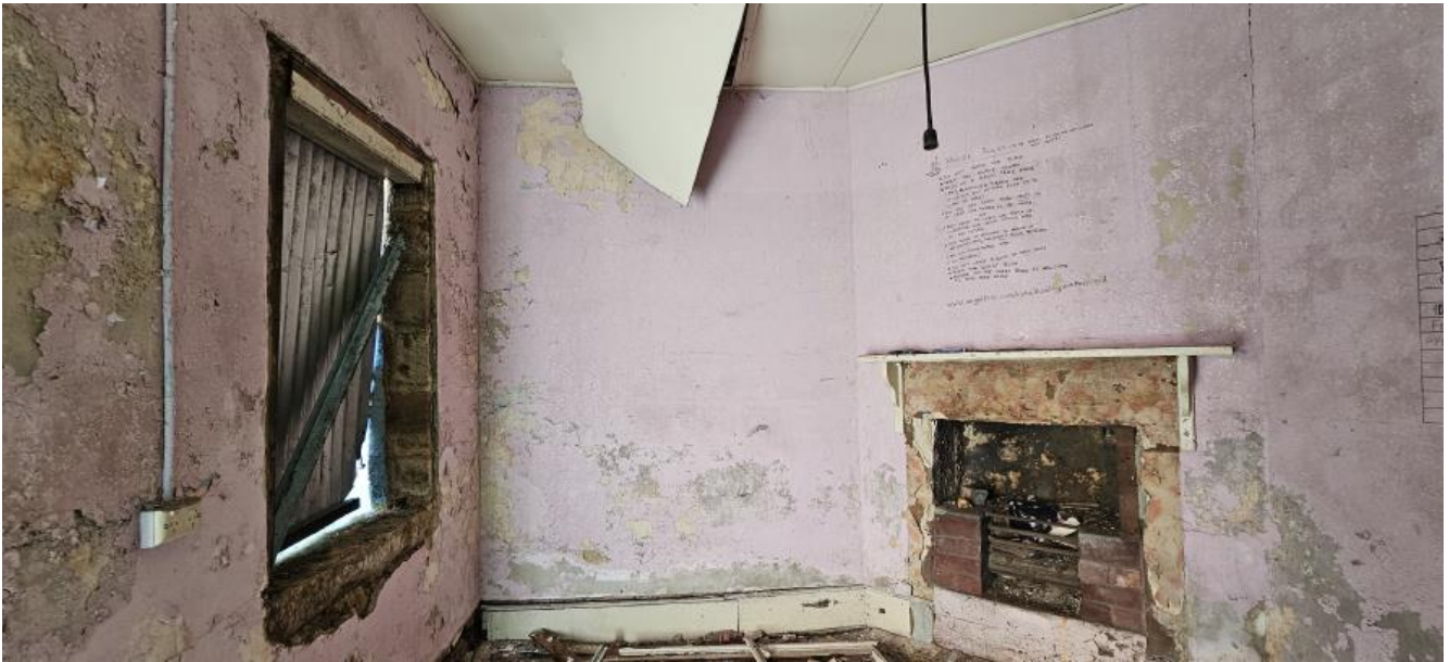
Figure 15: The rear north room
