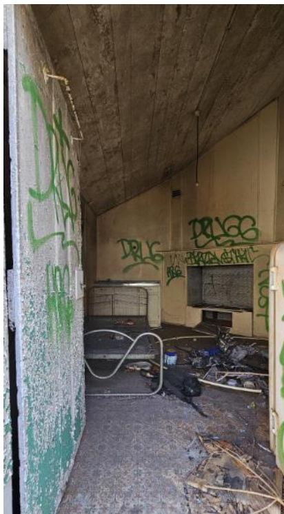
Figure 17: Interior of kitchen
