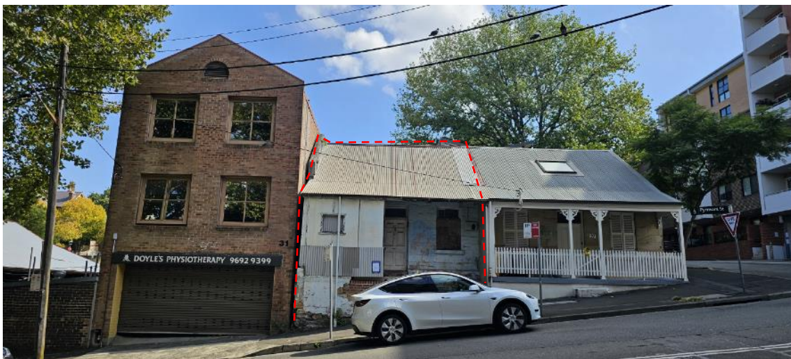
Figure 2: Site (outlined red) viewed from Pymont Street facing west
